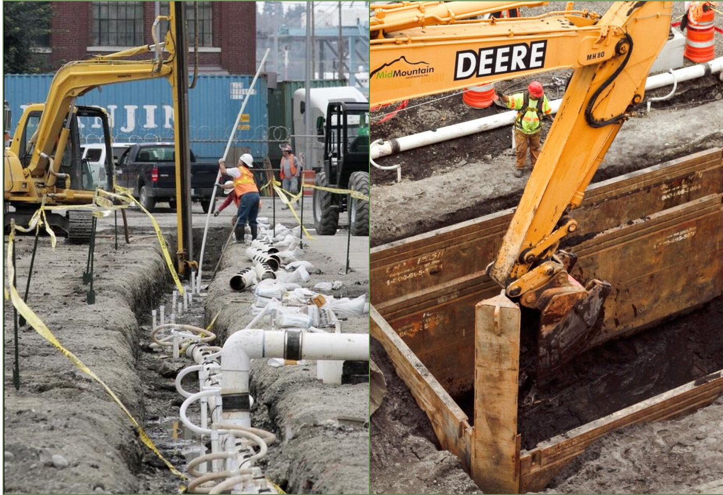
Crews are installing dewatering systems at several locations.
